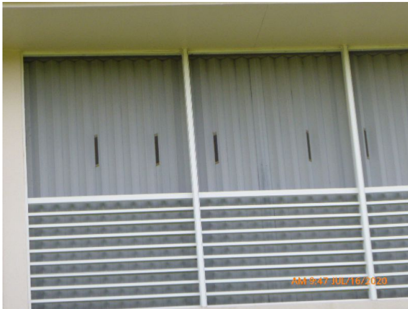
Accordion Shutter - Unverified as Impact
