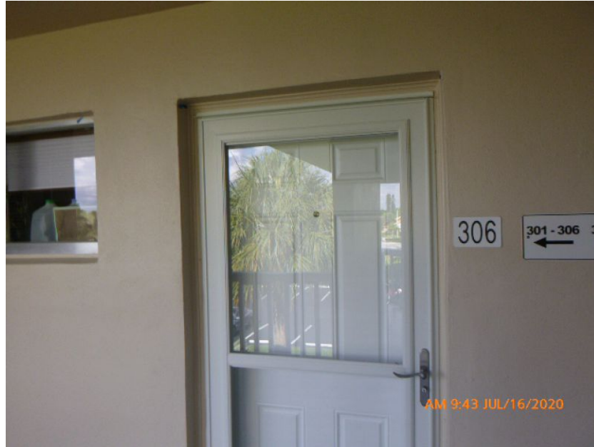
Unprotected Solid Entry Door
