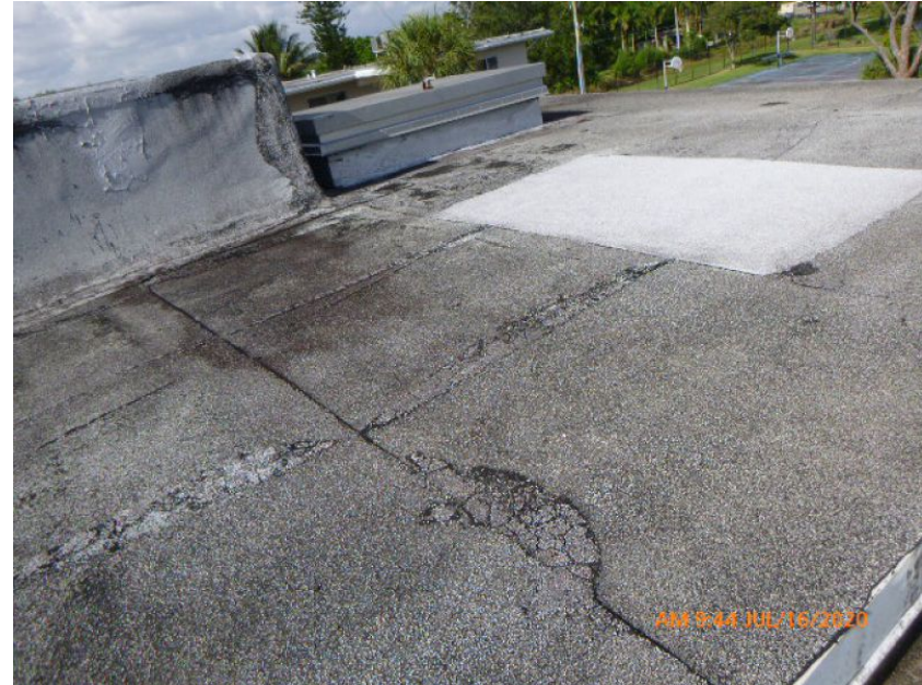
Built-Up/Rolled Asphalt Roof Covering
