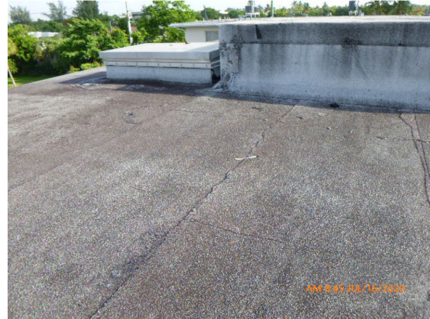
Built-Up/Rolled Asphalt Roof Covering
