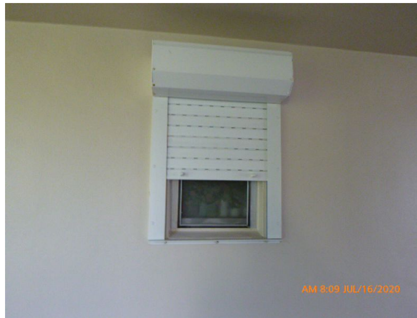
Non-Impact Rated Roll Down Shutter
