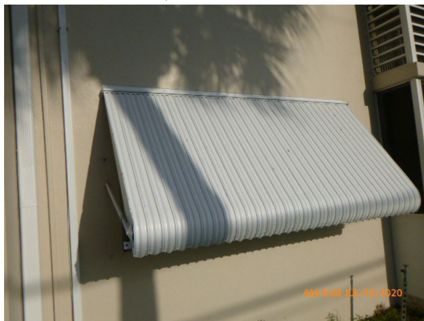
Non-Impact Rated Clamshell Awning Shutter
