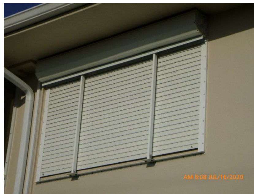
Non-Impact Rated Roll Down Shutter
