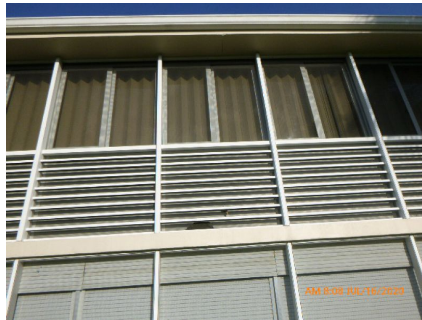
Non-Impact Rated Roll Down Shutter
