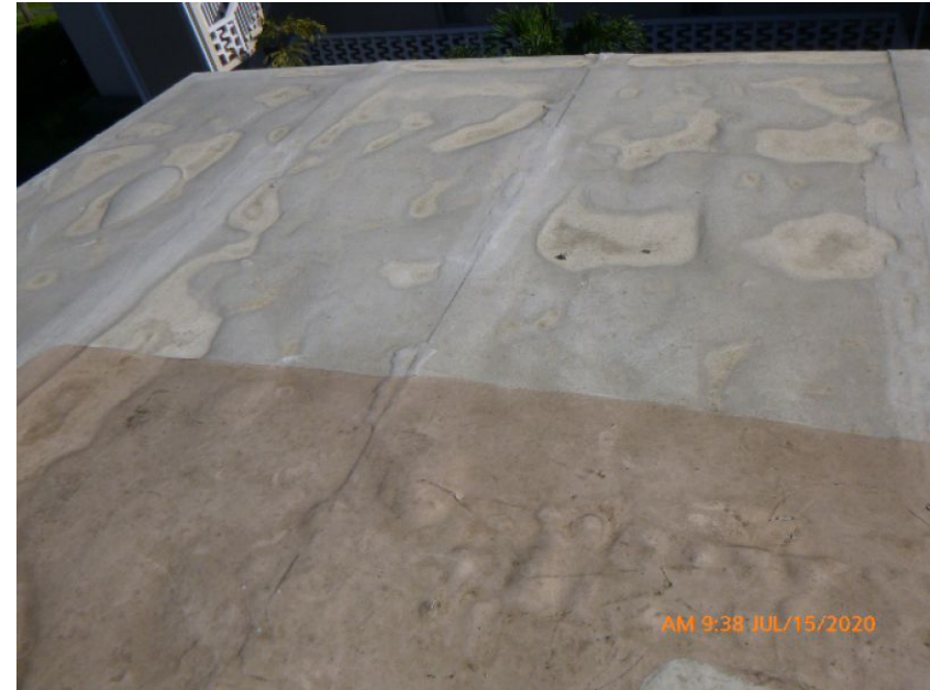
Built-Up/Rolled Asphalt Roof Covering
