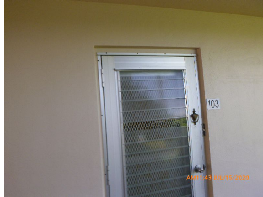
Unprotected Glazed Entry Door
