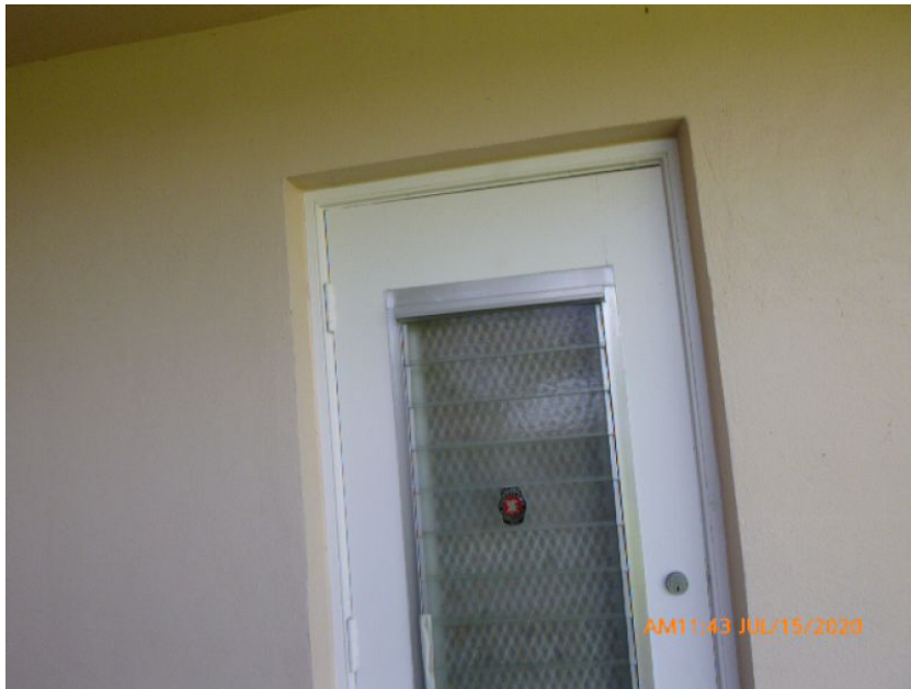
Unprotected Glazed Entry Door
