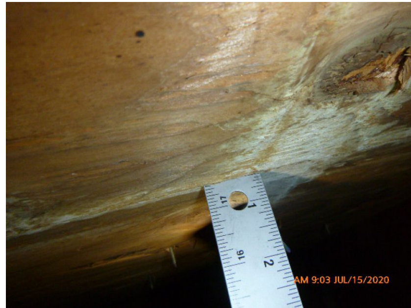
19/32" Deck Thickness Confirmed
