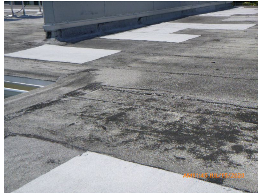
Built-Up/Rolled Asphalt Roof Covering
