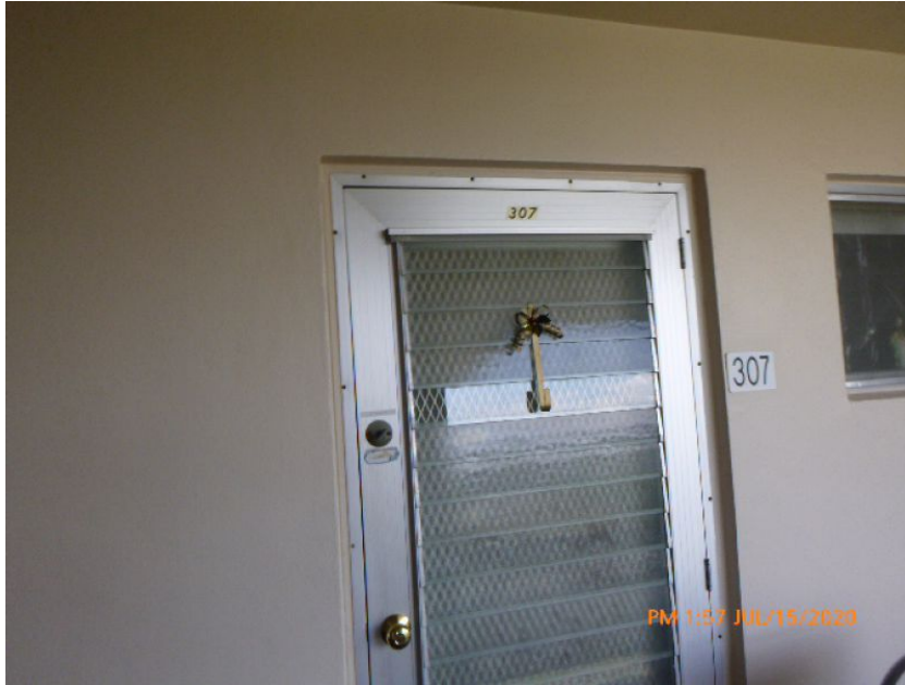
Unprotected Glazed Entry Door
