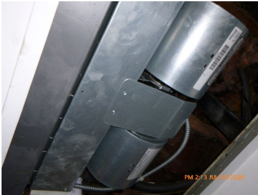
No Attic Access
