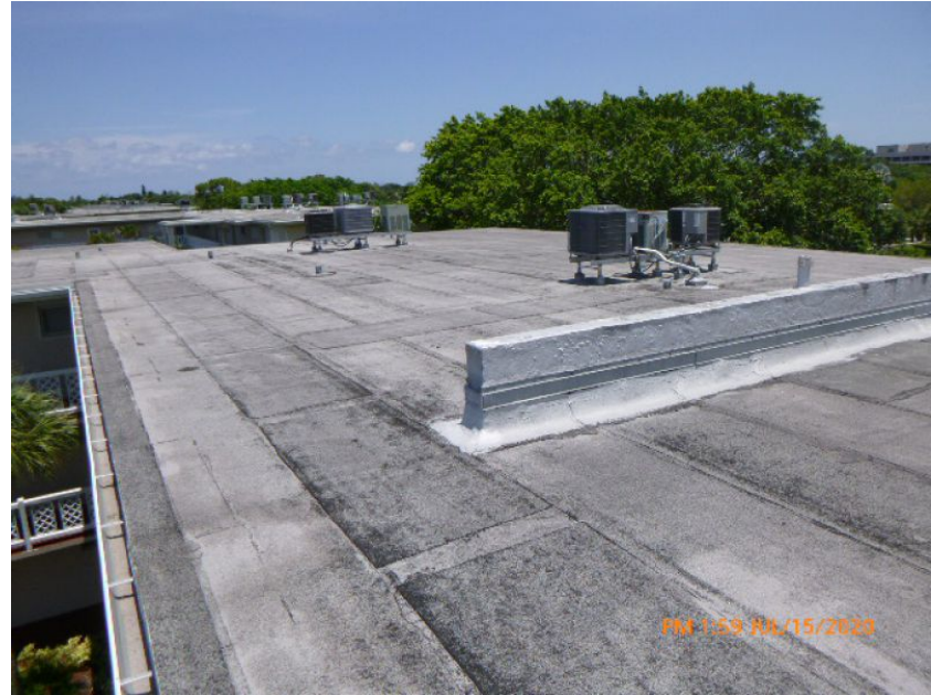
Built-Up/Rolled Asphalt Roof Covering
