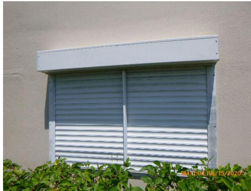
Non-Impact Rated Roll Down Shutter
