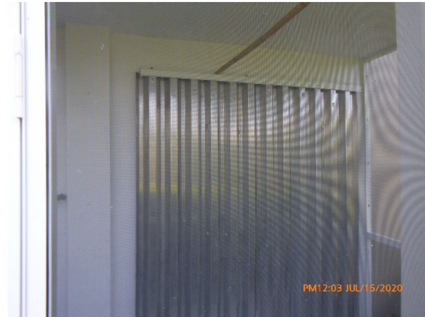
Panel Shutter - Unverified as Impact
