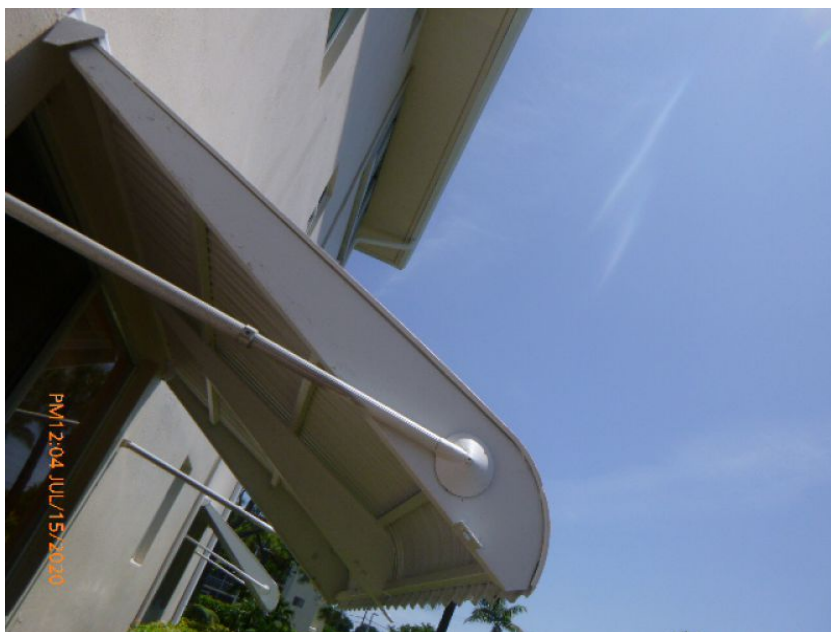
Non-Impact Rated Clamshell Awning Shutter
