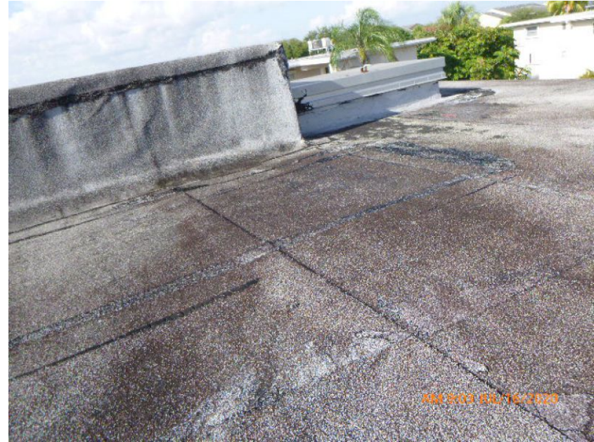
Built-Up/Rolled Asphalt Roof Covering
