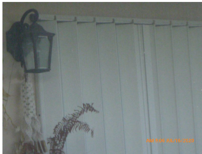
Non-Impact Rated Accordion Shutter
