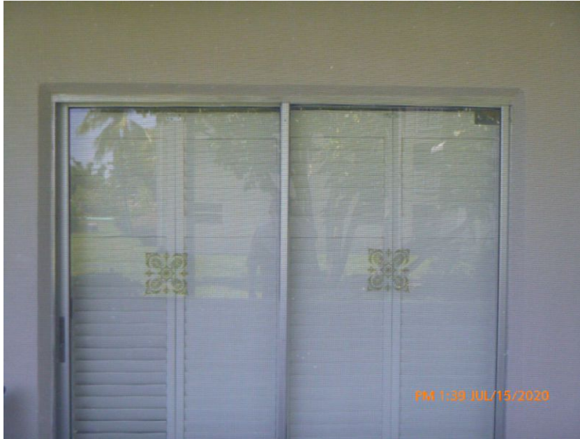
Unprotected Glazed Entry Door
