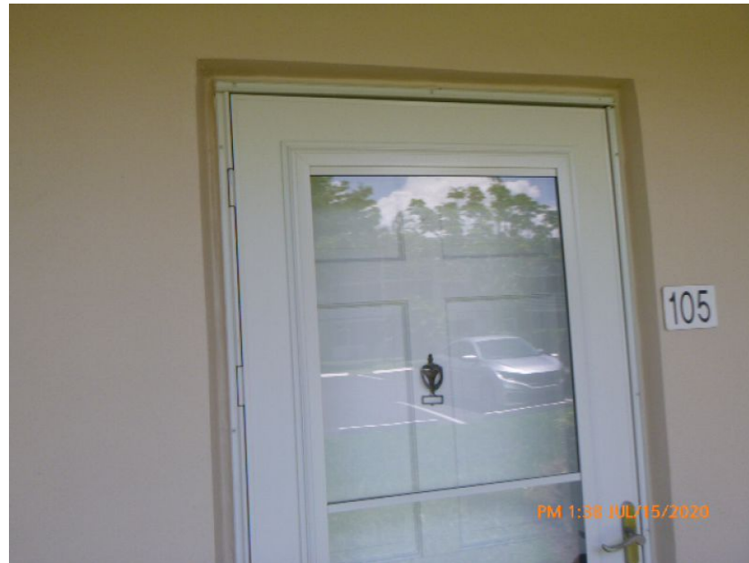
Unprotected Solid Entry Door
