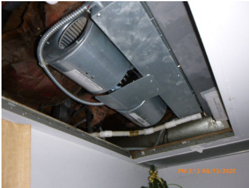
Attachment Unknown due to No Attic Access
