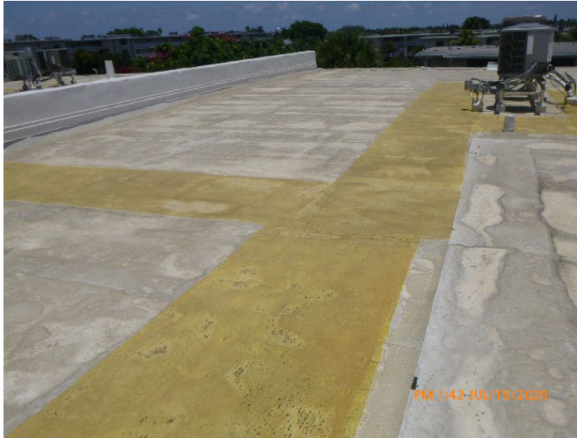
Membrane Roof Covering
