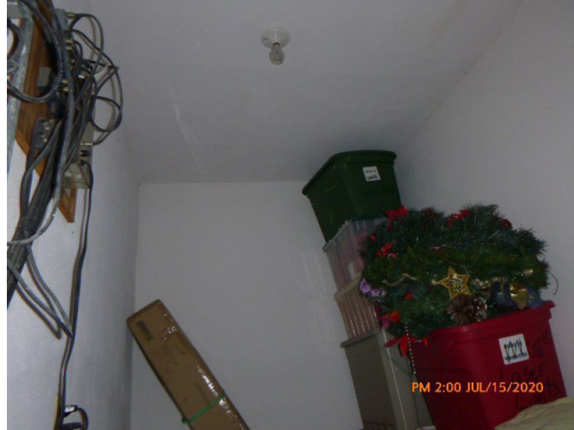
No Attic Access
