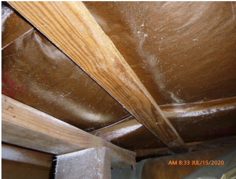
Attachment Unknown due to Insulation
