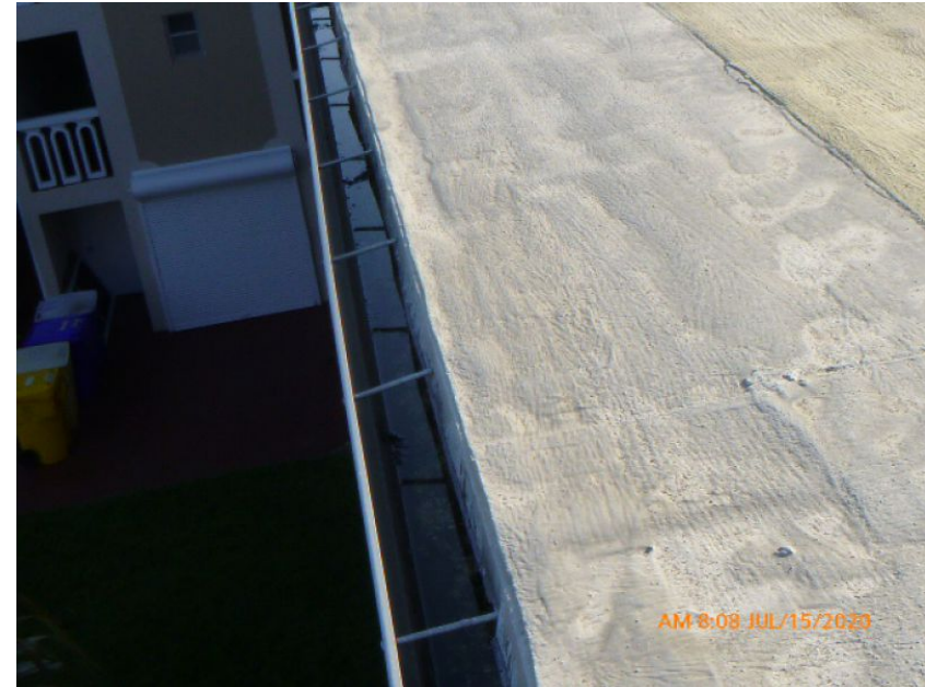
Built-Up/Rolled Asphalt Roof Covering
