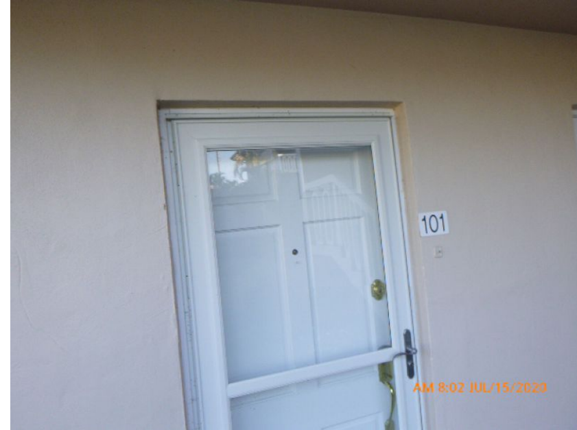
Unprotected Solid Entry Door
