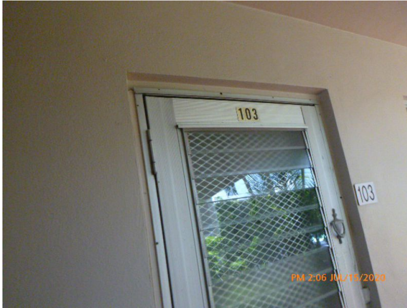
Unprotected Glazed Entry Door
