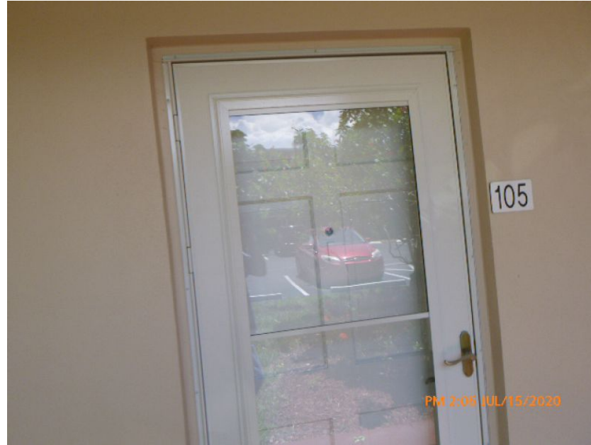
Unprotected Solid Entry Door
