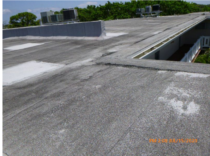
Built-Up/Rolled Asphalt Roof Covering
