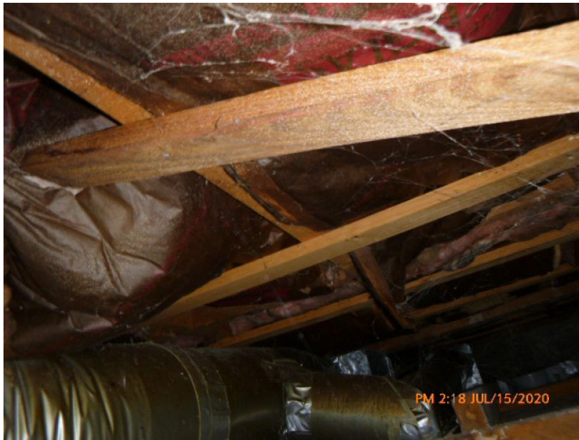
No Attic Access
