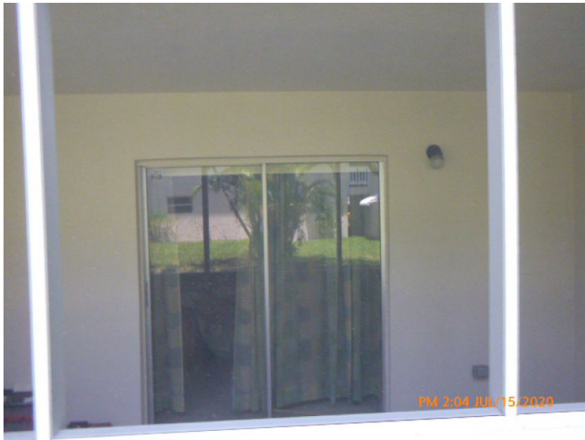
Unprotected Glazed Entry Door
