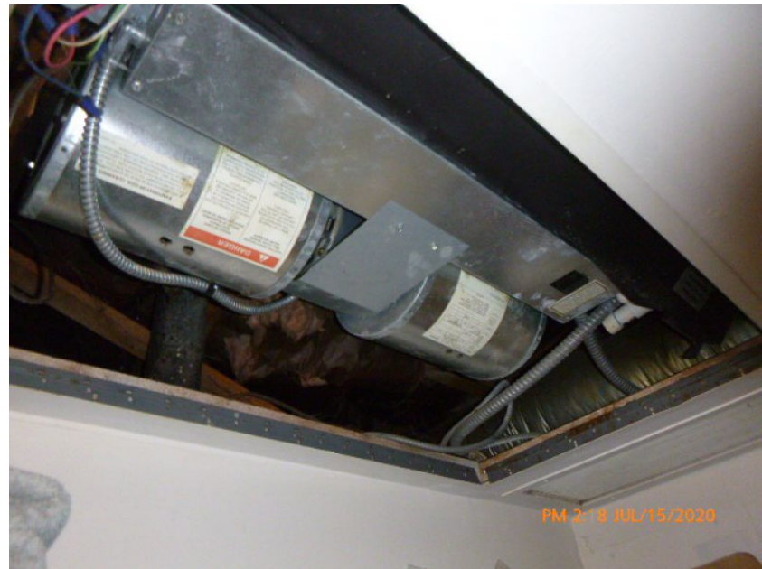
Attachment Unknown due to No Attic Access
